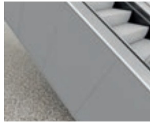
Grey powder coated sheet steel cladding (RAL7036) ***
